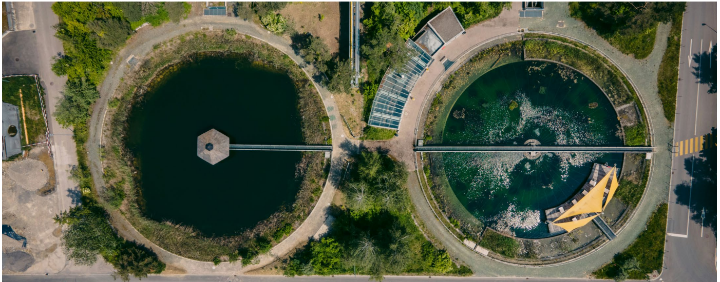
Wastewater treatment plants. Photo by Patrick Federi on Unsplash.
